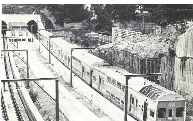
The above-ground section at Woollahra which is being restored by heavy planting of trees and shrubs.
