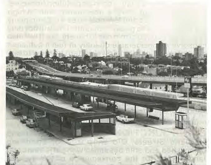
Bus deck above Bondi Junction Station nearing completion.
