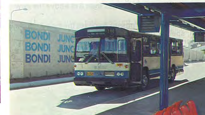
Section of the bus deck at the Bondi Junction Bus/Rail interchange complex.
