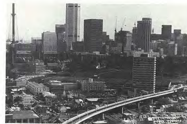
The ESR's Woolloomooloo Viaduct with the city skyline as a backdrop.
