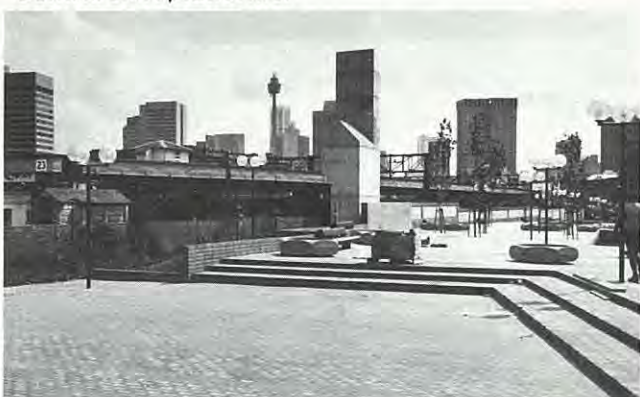
After — Restored Chalmers Street showing attractively landscaped pedestrian boulevard.
