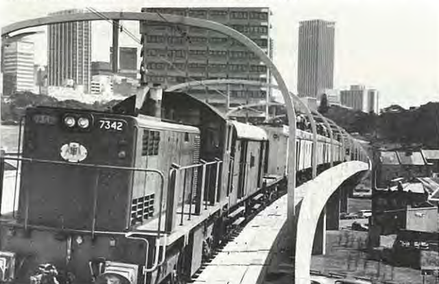
Overhead wiring train hauled by diesel-electric locomotive specially modified to eliminate harmful fumes.
